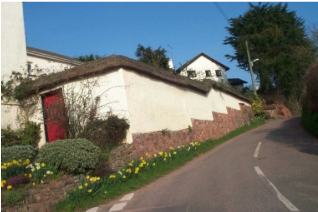
18. High walls with thatched coping
