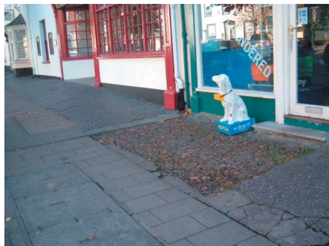
8 Damaged and obscured traditional surfaces
