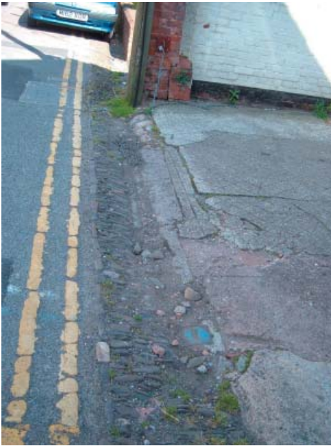
10 Damaged and obscured pebble lined gully
