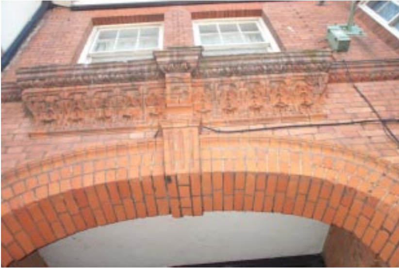
25. Moulded brickwork
