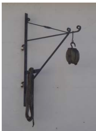
Figure 33 Hanging bracket and pulley at No 4 High Street
