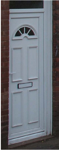
18 uPVC door with mock Georgian fanlight inserted in the door
