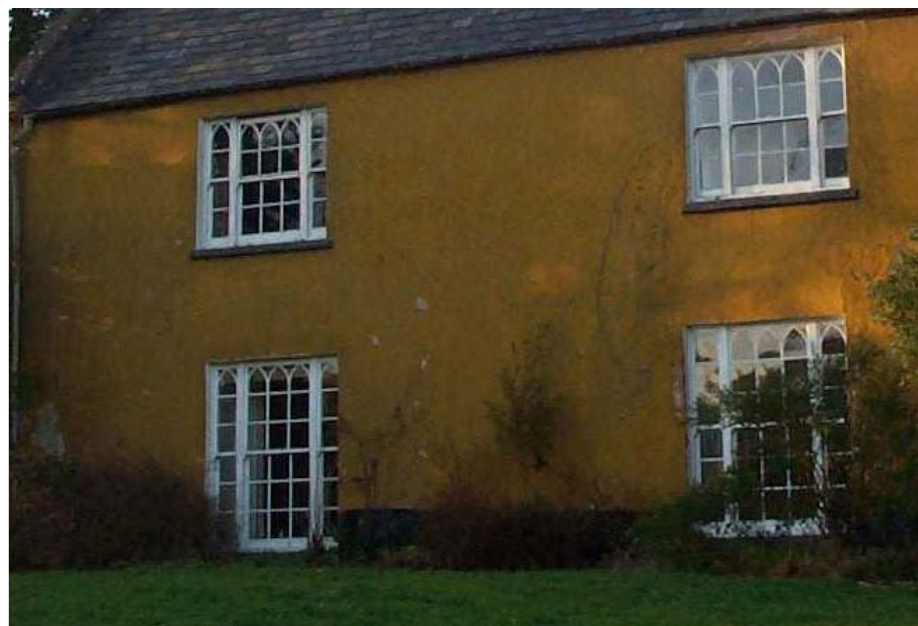
8 Vertical sliding sash with Gothic detail
