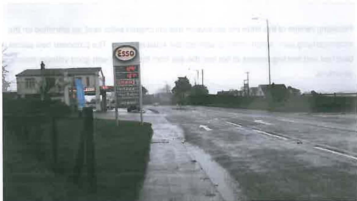
Access onto B3181 looking North East
