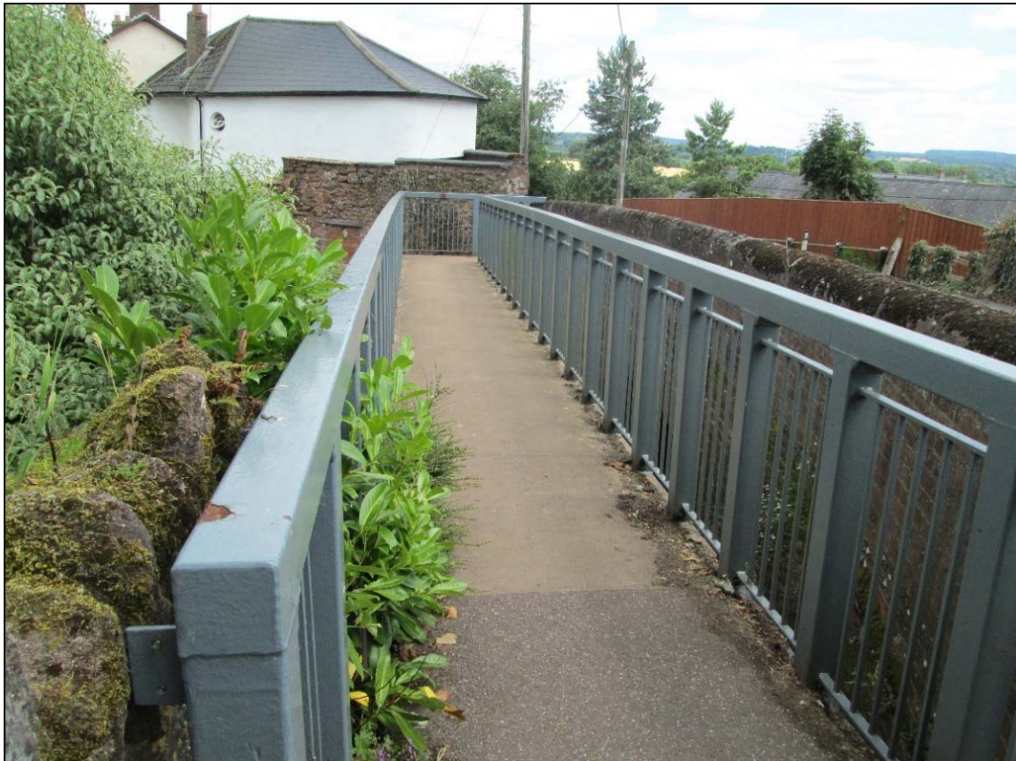
Figure 2 - Pedestrian Footbridge over the Canal (Higher Town / Turnpike / Lower Town)
