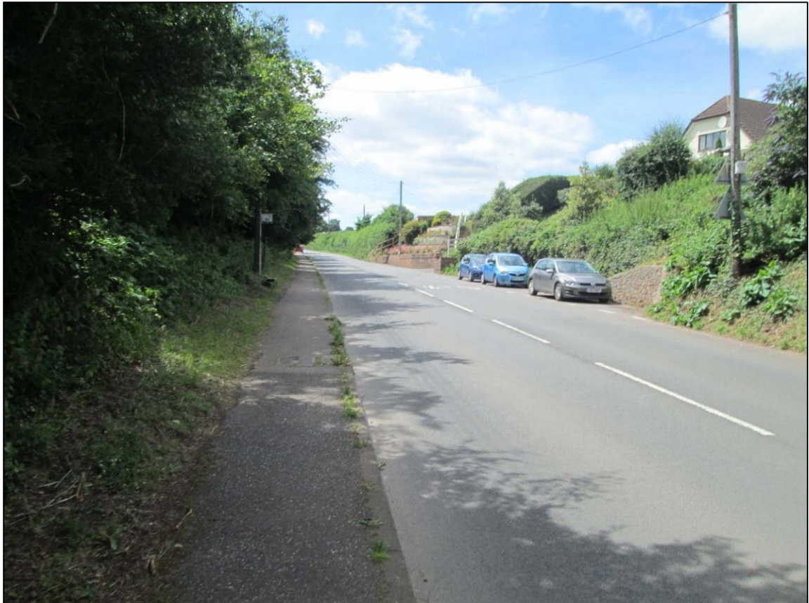
Figure 1 - Existing Footway along Turnpike (Orientated West Looking Towards the Site)
