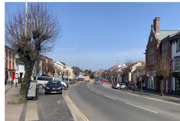
Above: View down the High Street in Cullompton
