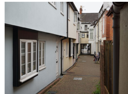
NETWORK OF YARDS AND PASSAGES Interesting and important network of yards and passages, reflecting former burgage plots.
