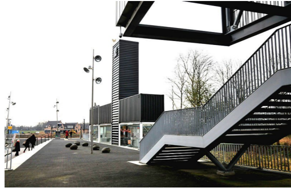
Figure 38 Barneveld Noord Station in the Netherlands uses shipping containers to make a very light touch and cost effective facility. Image Copyright: Spoorjan, CC BY-SA 3.0 < https://creativecommons.org/licenses/by-sa/3.0/ >, via Wikimedia Commons
