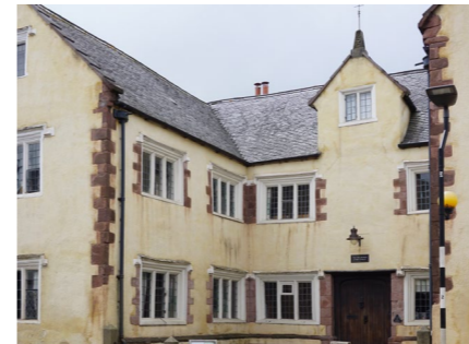
OUTSTANDING BUILDINGS Some outstanding buildings especially St. Andrew's Church and the Walronds
