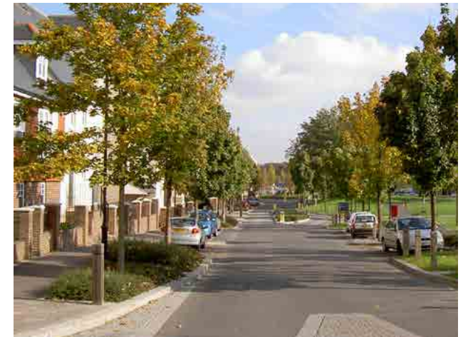
↑ Example of a single-sided residential frontage orientated to overlook a parkland
