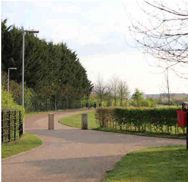
↑ Example of a self-binding gravel pathway adjacent to existing and new planting
