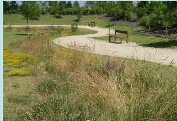
↑ Example of landscaped swale and sustainable urban drainage feature that supports water-saving measures.
