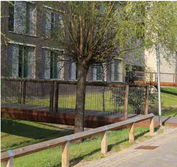
↑ Pedestrian bridge spanning a swale, providing access to a residential plot
