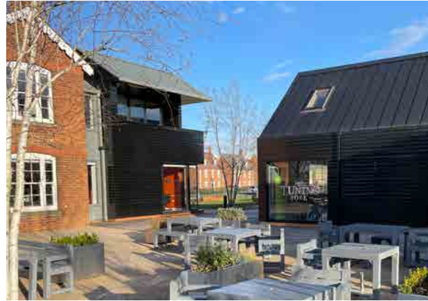
↑ Example of existing buildings being used as a hub of activity and place to meet
